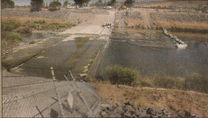
The Alameda County Water District is modifying the foundation of a rubber dam along Alameda Creek in Fremont to allow fish to pass through the area under low-flow conditions.
